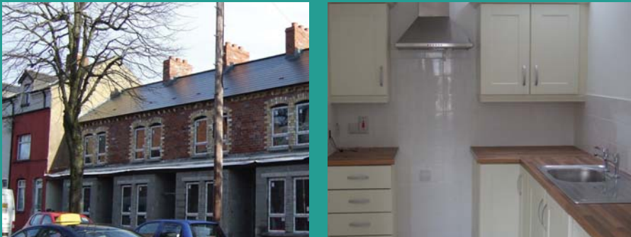
Village Rehabs. Donegall Road external and internal views
