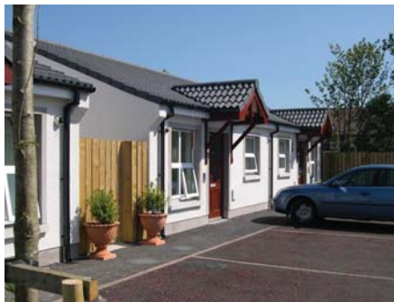
Habinteg Housing development at Hillmount Court, Finaghy South Belfast
