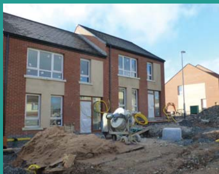
Andersonstown Library Site: new build under construction
