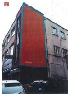
2 End wall facing down Church Lane
