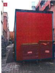
1 Gable wall perpendicular to Church Lane
