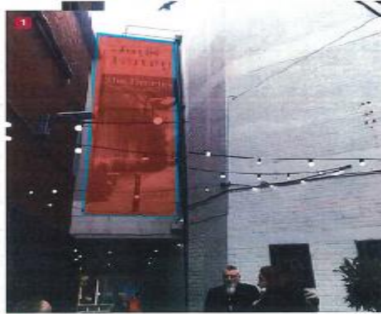
1 Ann Street overhang face and adjoining wall
